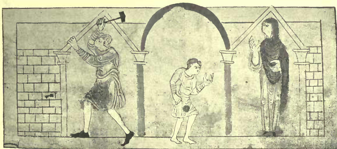
CRAFTSMAN AT WORK ON A HOUSE
